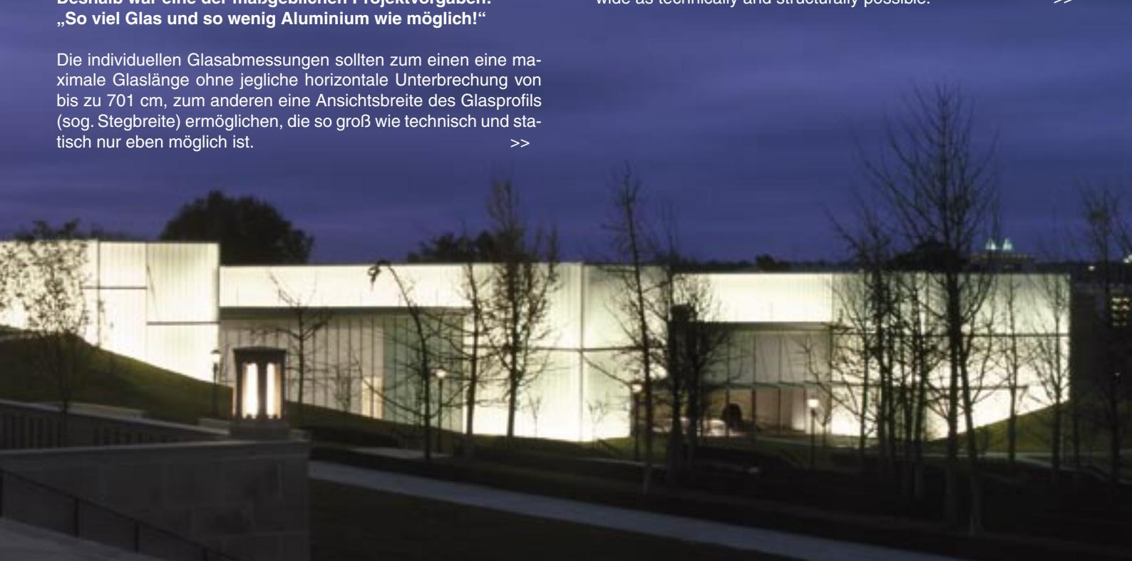
Owing to a solar texture on the outer surface of the channel glass and the sandblasted inner face of this outer wall, the exterior takes on an opalescent sheen in sunlight, rather like chantung silk. Although it sometimes appears flat in even light, as exterior conditions change, a glinting moiré pattern emerges.
